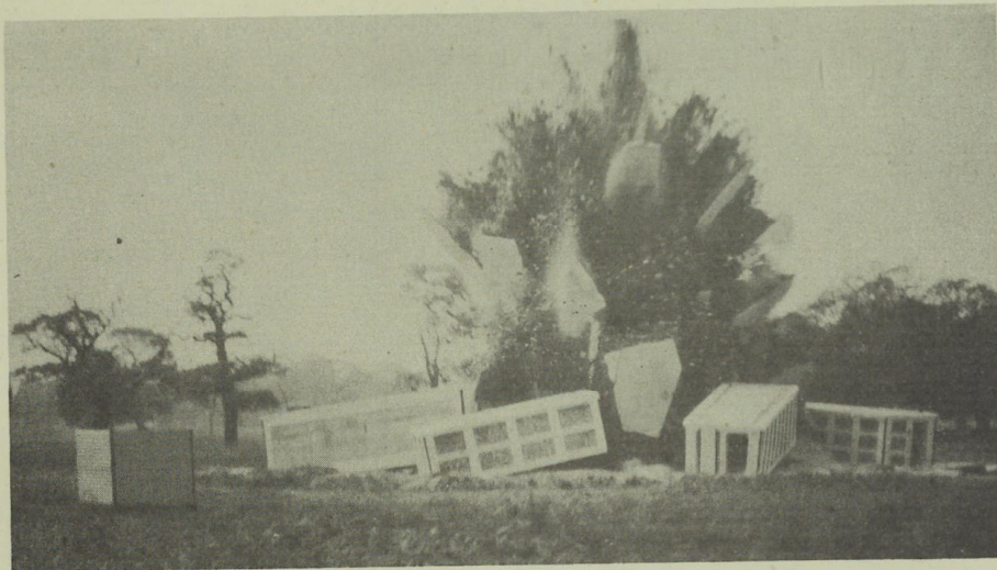
Fig.8.7 Effect of ground-shock on a group of reinforced brick surface shelters and one reinforced concrete shelter (on extreme left). Note how shelters are thrown into the air without fracture. (Paragraph 8)
